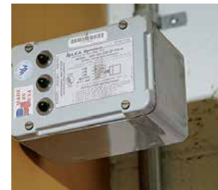
Surge protector mounted at the electrical panel.
