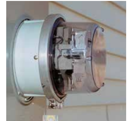
Surge suppressor mounted behind the meter.
