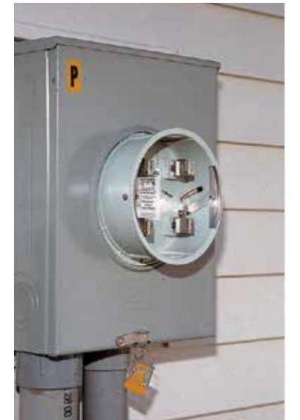
Surge suppressor mounted near the electrical source.
